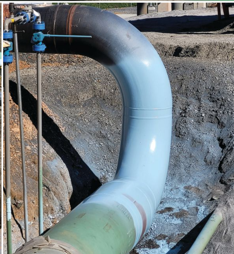
Over the course of 9 months, M J Painting had to abrasive blast and coat the 25,000–30,000 square feet for above- and below-ground areas.
