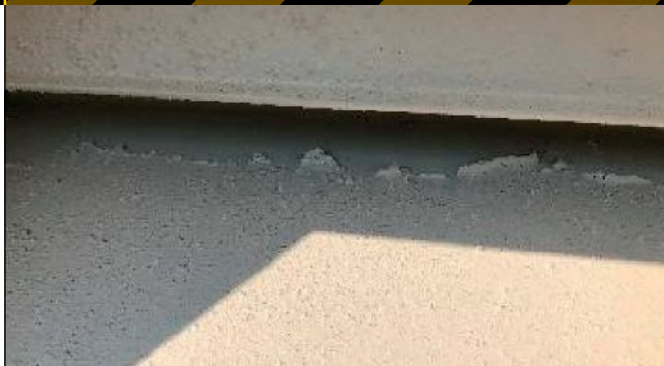
No cleaning or surface preparation done prior to applying the paint
