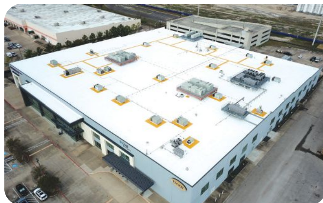
The last step was to install two coats of yellow AcryLink G at an average of 40 mils DFT each with EPDM granules broadcast into the first coat.
