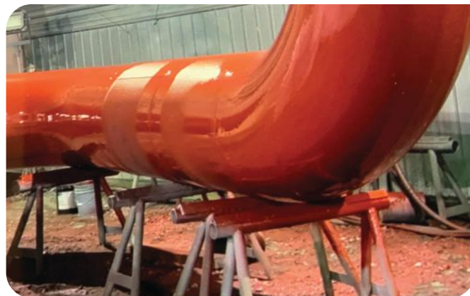
Below-ground areas received 20–50 mils DFT of SPC SG-2888 RC, and above-ground areas received 12–18 mils DFT of epoxy. Tie ins were coated after the equipment was installed.
