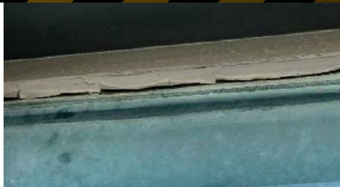
Delaminating paint visible
