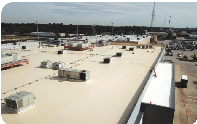
The crew applied two coats of AcryLink G at an average of 15 mils DFT each, and rolled areas that couldn't be sprayed.
