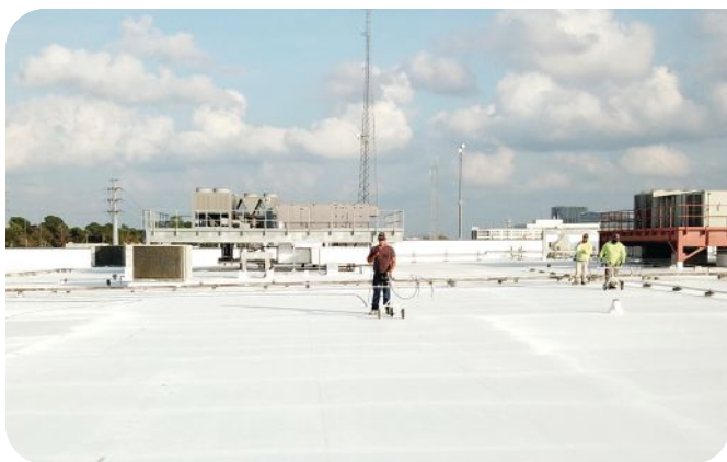
The crew used an ELD device on each of the roof's sections to identify and chase and leaks, punctures, and penetrations.
