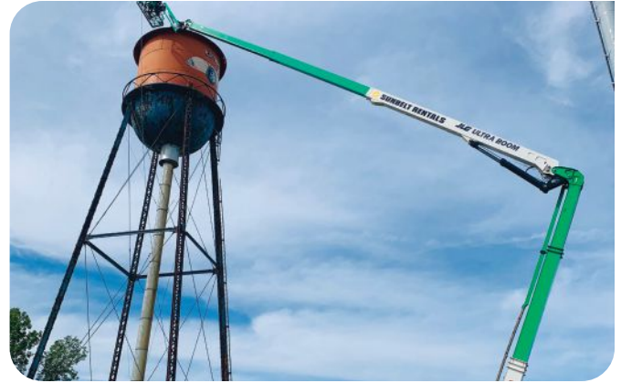
They started by working from a 160-foot boom lift, wearing harnesses as well as other PPE.
